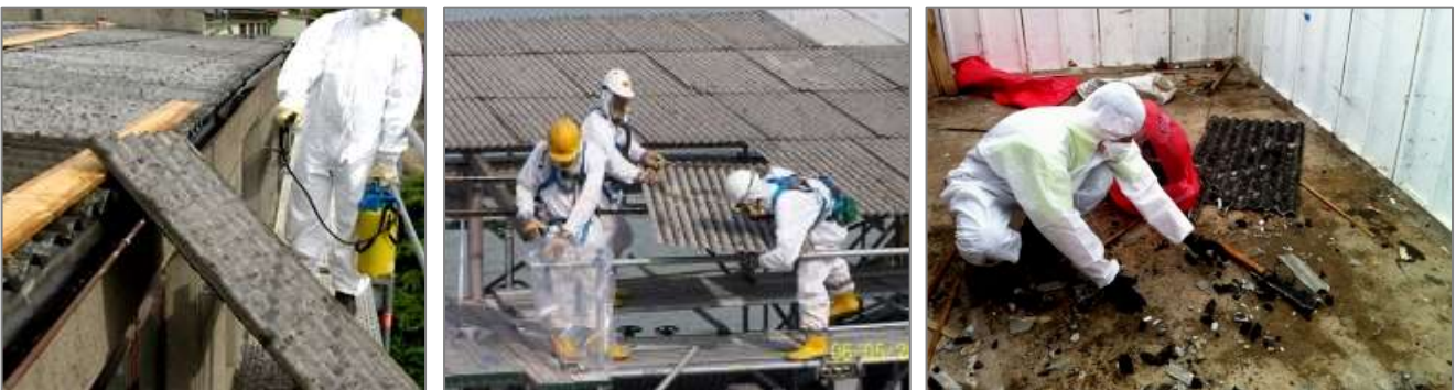
Figure 7 – Safe removal of asbestos cement roofing sheet and debris
