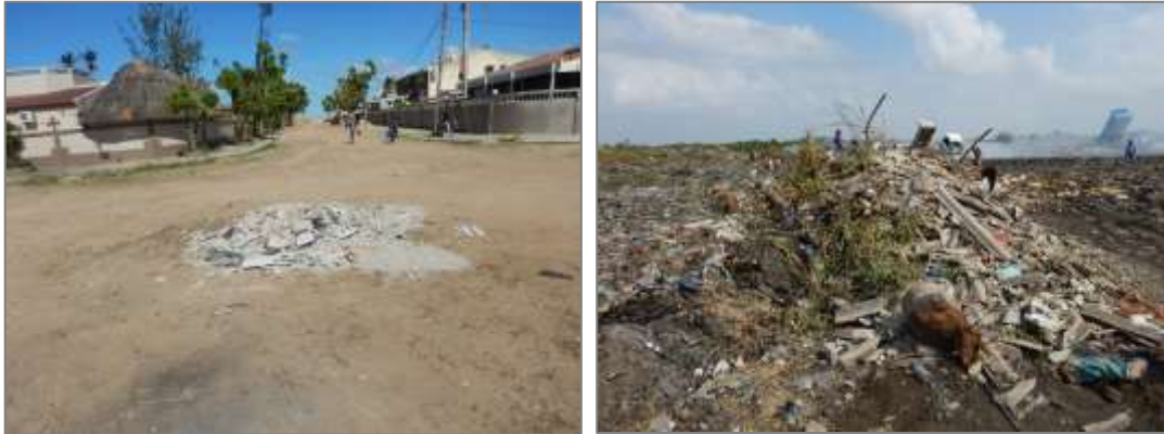
Figure 3 – Filling of potholes with asbestos cement rubbles and disposal at Beira dumpsite
