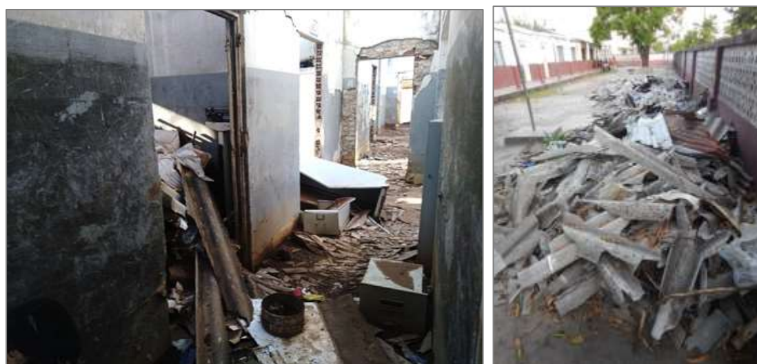
Figure 2 – Asbestos cement debris among rubbles in Buzi rural hospital (left) and in Beira city (right)
